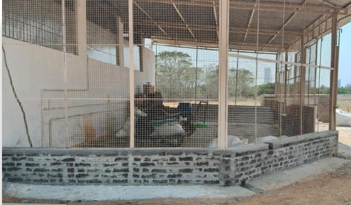
Material Recovery center Bangalore 4,000 Wricks 6 Months
