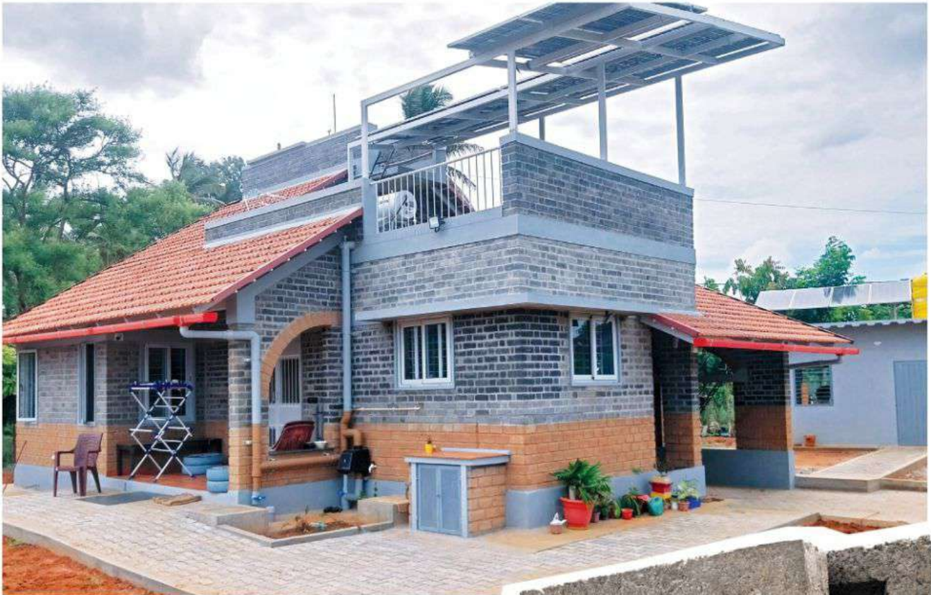
Wricks® offers strength, waterproofing and insulation while fitting into existing construction practices.
